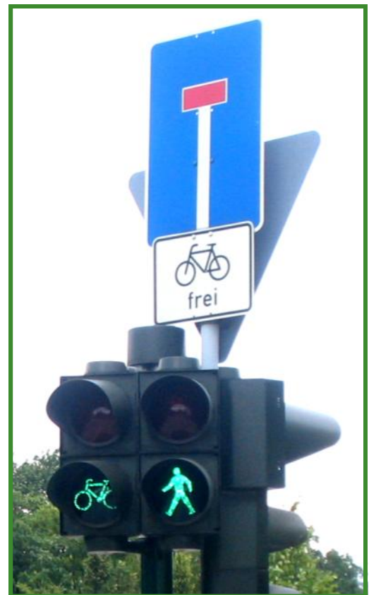
▲ Bicycle and pedestrian signal head
