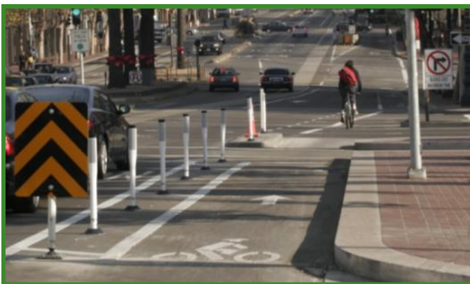
▲ One-way barrier-separated bike lane
