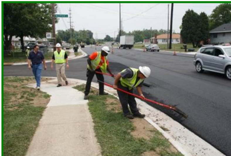
▲ Rubberized Asphalt (Photo: Franklin County Engineers Office)
