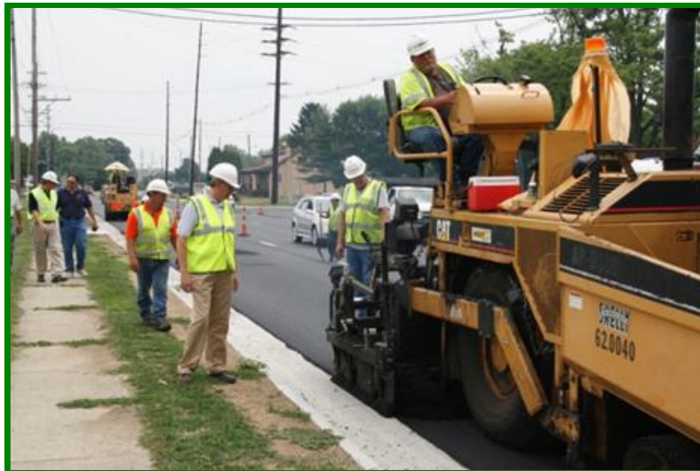
◀ Rubberized Asphalt (Photo: Franklin County Engineers Office)
