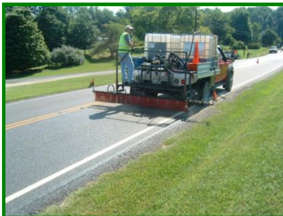
◀ RePlay being applied to a road in Licking County, Ohio (Photo: Ohio Pavement System)
