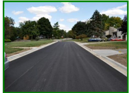
▲ Edgevale Road after the Greenroads process (Photo: Upper Arlington, Ohio)
