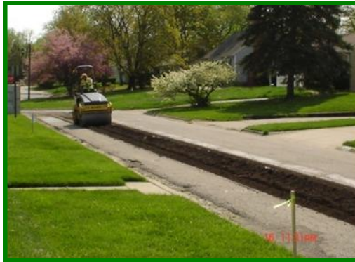
▲ Edgevale Road during the Greenroads process (Photo: Upper Arlington, Ohio)
