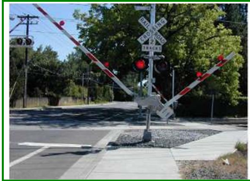
▲ Example of a pedestrian crossing at a railroad with gates and lights. (Photo: FHWA)
