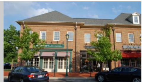
Example of commercial buildings under form-based code in New Albany. (Source: MORPC staff)
