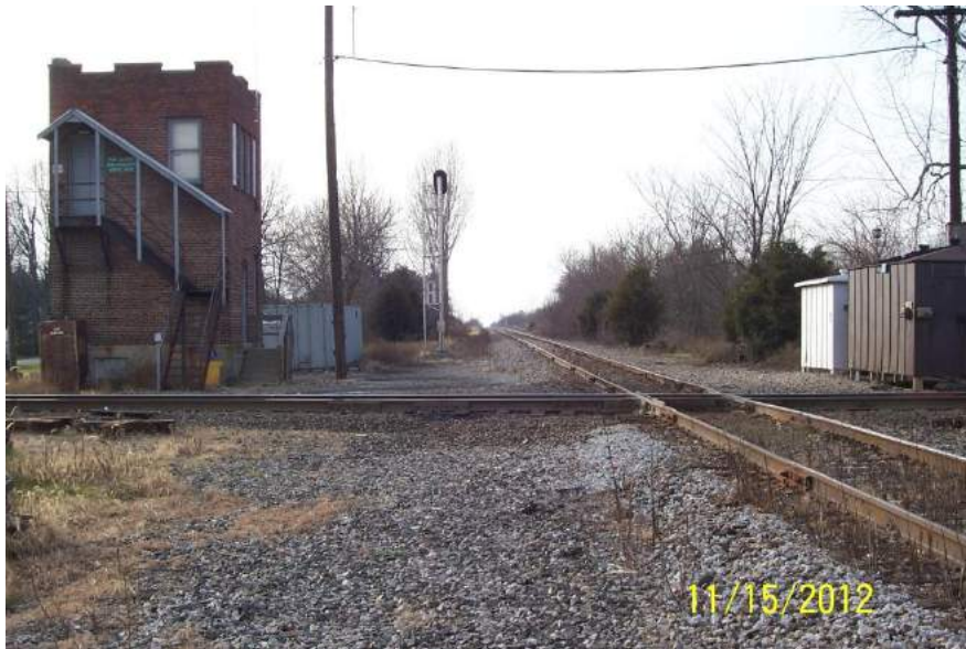
Photo 9: Dunkirk Crossing looking West on the Fort Wayne Line. The passenger train would switch off onto a high-speed connection track before it reaches this point.
