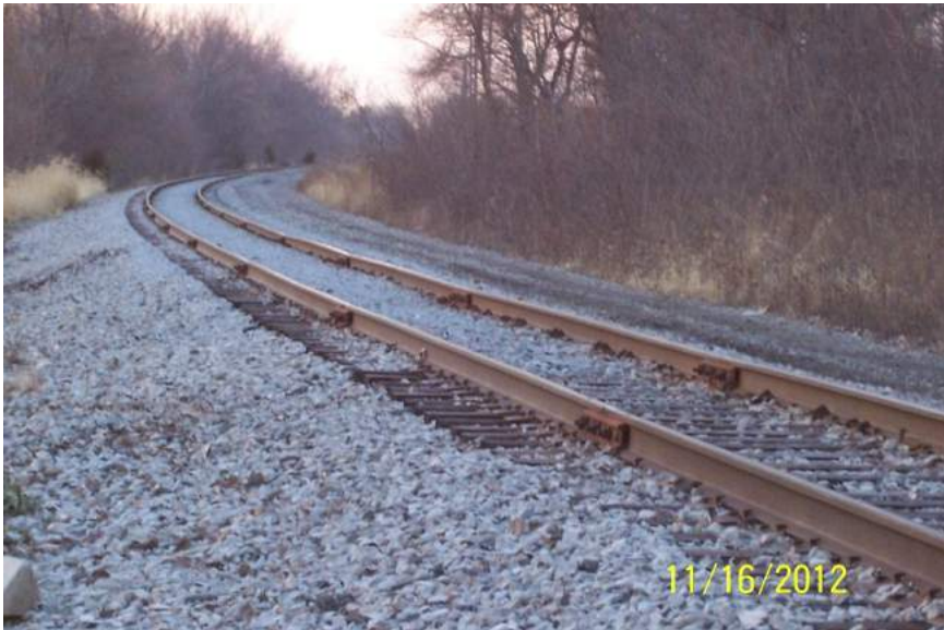
Photo 29: 2° 06' Curve at MP 435.3 at Hobart.
