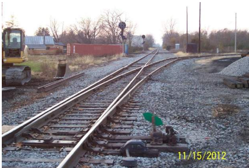
Photo 19: Branch line connection and Crossing Diamond in Van Wert, OH
