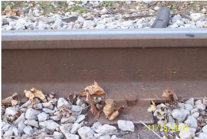
Photo 12: PRR #155 Jointed Rail still in service at Dola, Ohio
