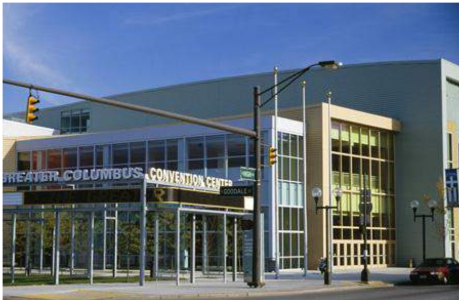
Photo 1: Planned Platform Area underneath Columbus Convention Center, showing Buckeye Line Junction at CP-138
