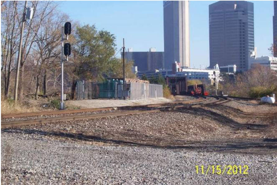
Photo 2: NS Dayton District Scioto River bridge
