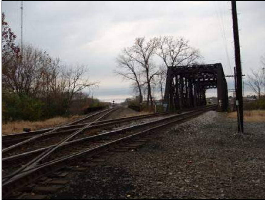
Photo 4: CP Hocking view west along the Buckeye Line. The double-tracked CSXT Columbus Subdivision to Marion passes through the girder bridge on the right.
