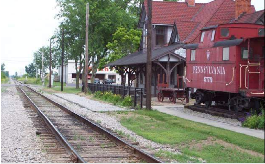
Photo 13: Fort Wayne Line at Ada historic passenger station MP 245.5 - View east
