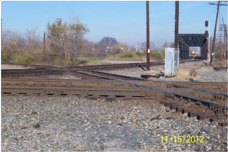
Photo 3: CP Scioto Diamond Crossing with Southbound CSX Train approaching on former C&O Columbus Subdivision
