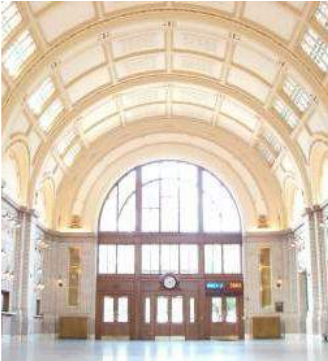
Photo 24: Interior of the restored Fort Wayne train station
