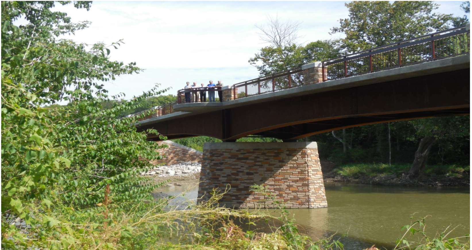
New trail bridge over the Great Miami River
