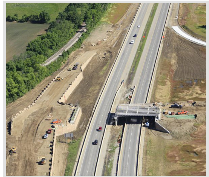
Construction of the recently completed Carroll Interchange at the south end of the corridor
