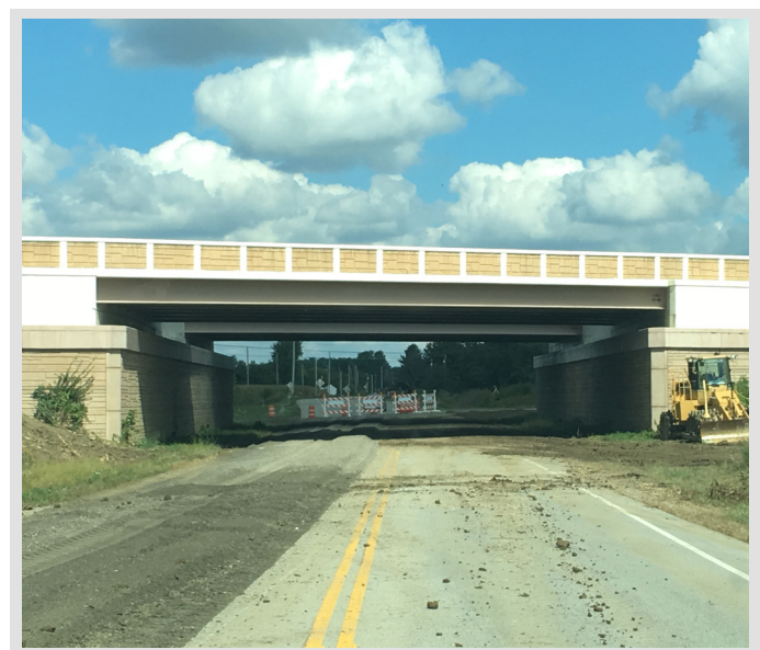
Construction of the new Mink Street Interchange with SR 161
