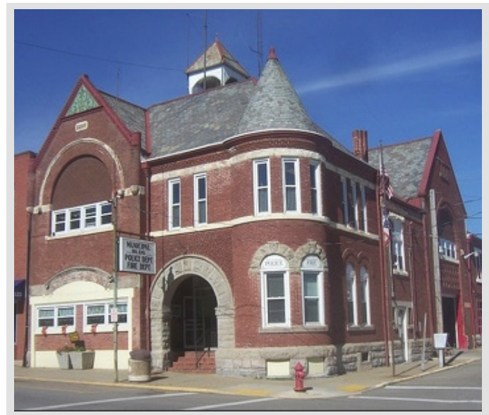
Former Town Hall and Opera House in New Lexington
