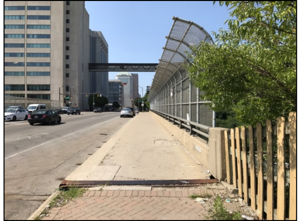
Figure 13 - High Street Bridge on eastern sidewalk of bridge (existing).
