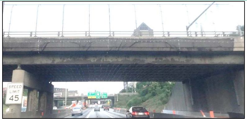
Figure 8 - Fourth Street Bridge current conditions.
