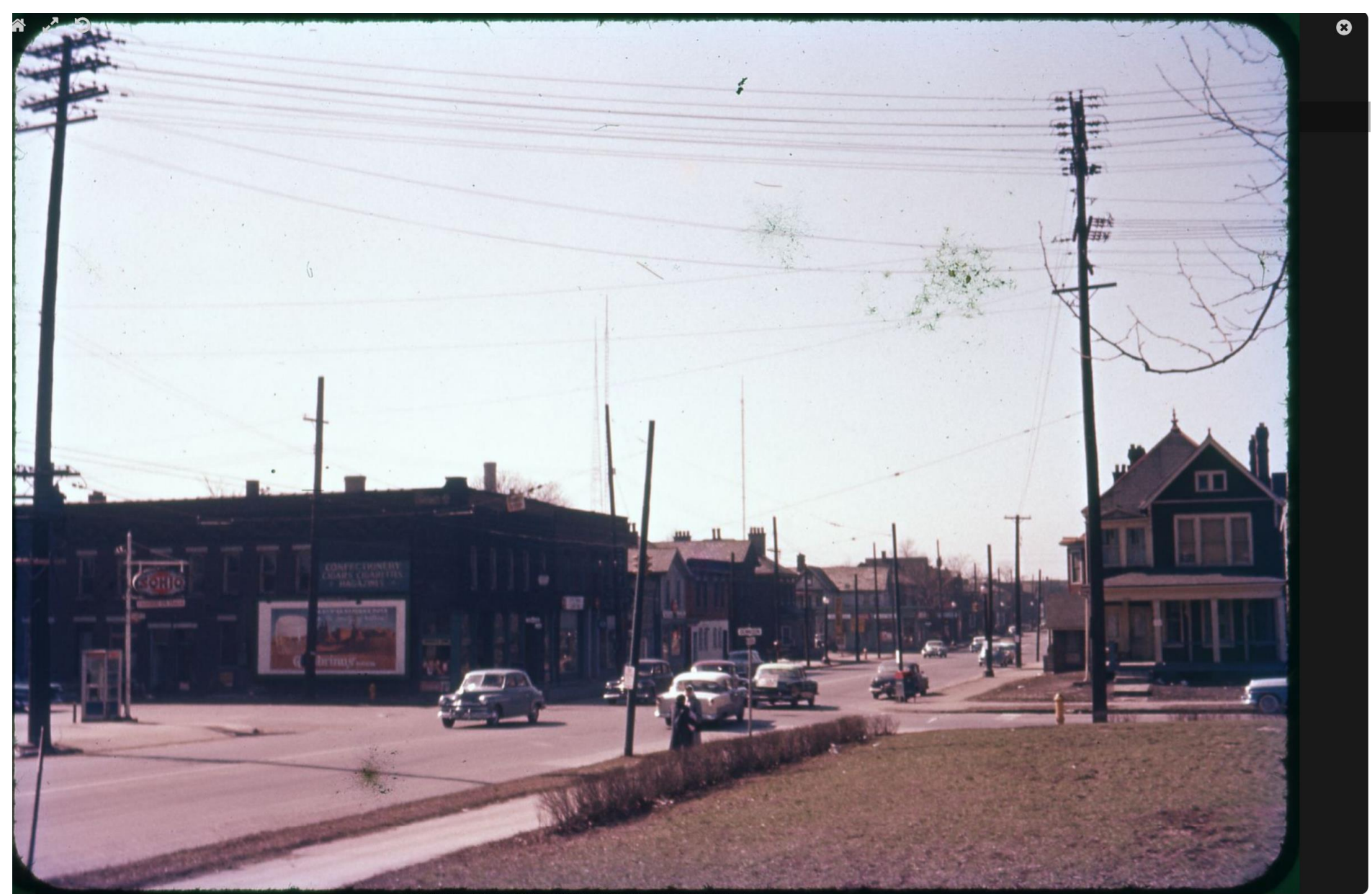
Flytown: Looking southwest from Goodale Park at the intersection of Goodale and Dennison March 3, 1957 (prior to construction)
