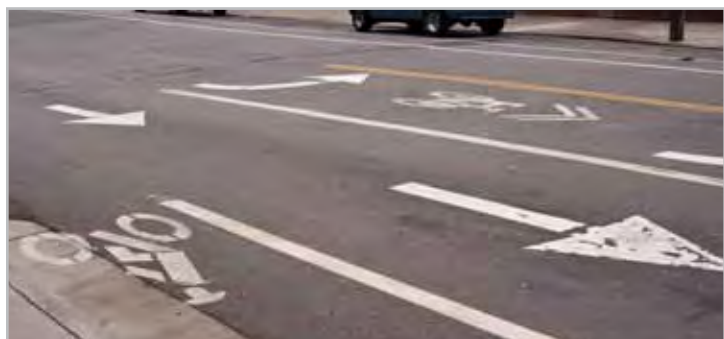
In addition to a bike lane for through traffic, the sharrow in the left turn lane encourages bicyclists to use the lane for left turns, and alerts motorists that bicyclists use the lane. The bike lane should not be in the gutter pan; otherwise, this is a good example. Source: Flickr/ sfbike. Portland, OR.
