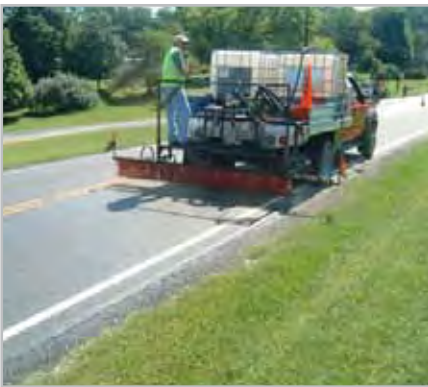
Replay is being applied to a county road. Source: Ohio Pavement Systems. Licking County, OH.
