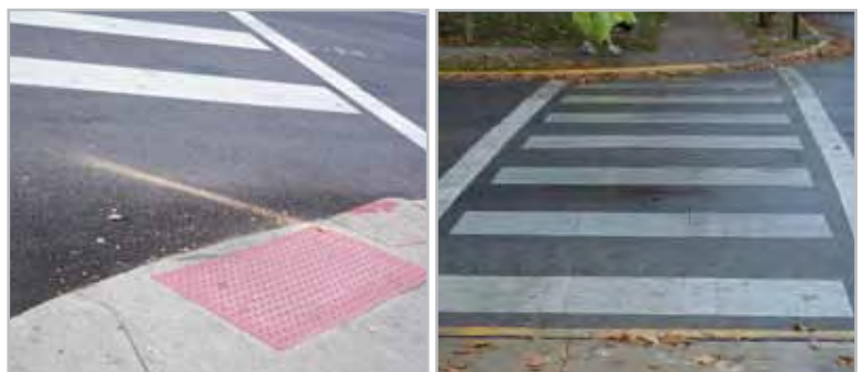
Left: ADA-compliant curb ramps. Right: This crosswalk lacks curb ramps, and therefore does not meet ADA requirements. Source: MORPC. Columbus, OH.
