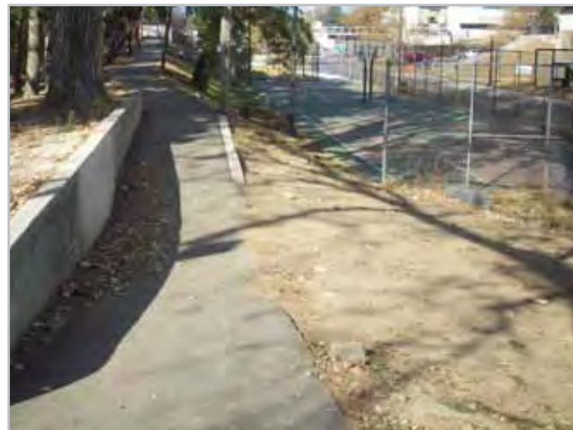
This MUP is too narrow to be used comfortably by multiple users. Source: MORPC. Columbus, OH.
