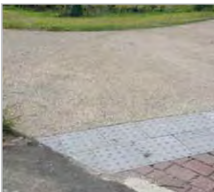
Pervious Pavement used as part of a parking lot. Source: Grange Insurance Audubon Center. Columbus, OH.
