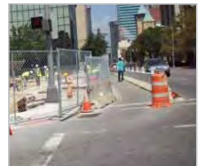
A travel lane was converted to a walkway during construction. Source: MORPC. Columbus, OH.
