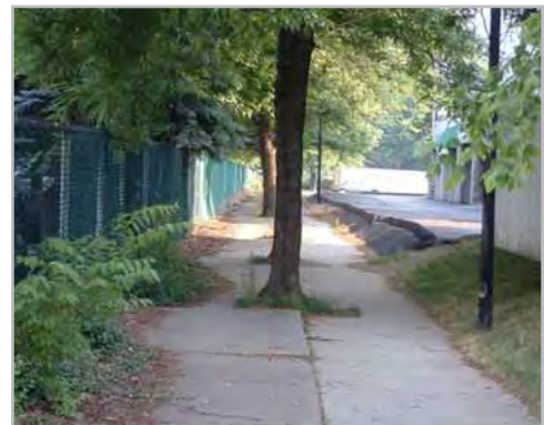
This tree blocks the sidewalk and has caused the sidewalk to heave. Source: MORPC. Columbus, OH.
