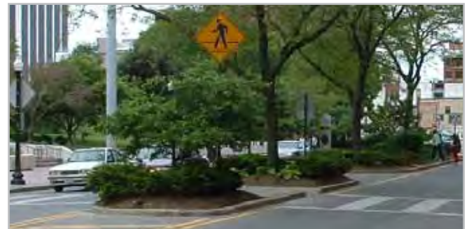
Pedestrian refuge islands break long crossings into two more manageable crossings. Source: MORPC. Columbus, OH.
