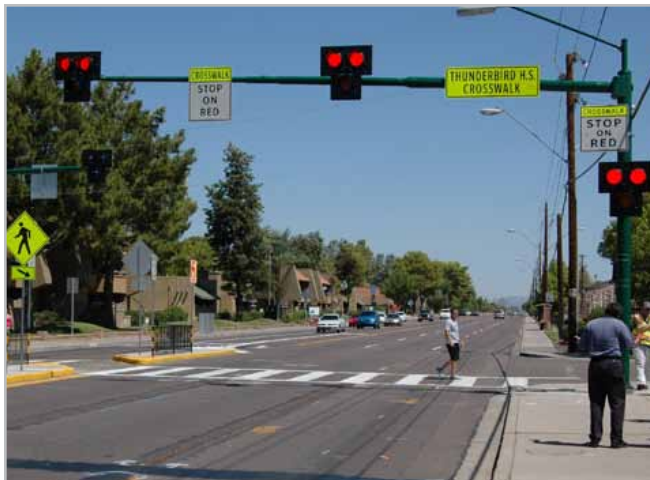
The HAWK signal gives a clear indication to motorists to stop for pedestrians. Source: Mike Cynecki. Phoenix, AZ.
