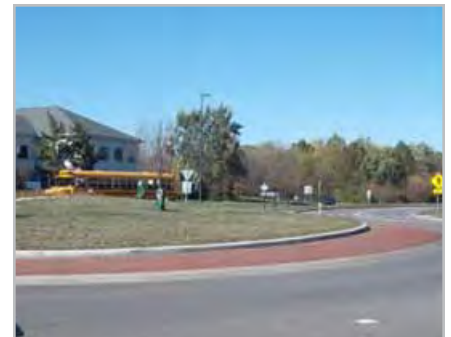
One-way Roundabout. Source: City of Dublin, OH.
