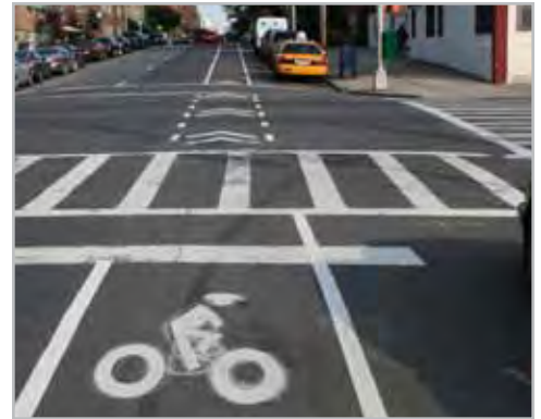
Extra space has been provided to reduce the chance of a car door opening into the bike lane. Source: WikiMedia. New York, NY.
