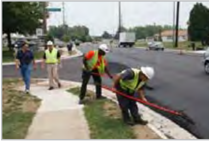
Rubberized asphalt installation. Source: Franklin County Engineer's Office, Franklin County, OH.
