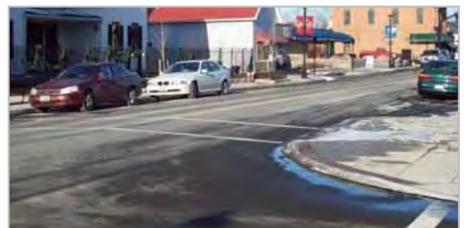
Curb extensions shorten the crossing distance, reducing pedestrian exposure. Source: MORPC. Columbus, OH.
