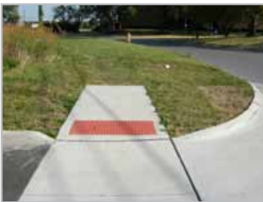
This sidewalk terminates abruptly, leaving pedestrians to walk in the grass or street. Source: MORPC. Columbus, OH.
