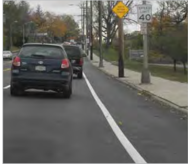
This bike lane has sufficient width for safe and comfortable riding and there are no gutter openings in the bike lane. Source: MORPC. Columbus, OH.
