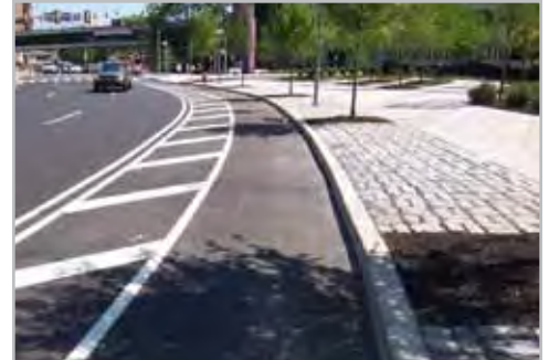
This contraflow bike lane provides two-way bicycle traffic on a one-way street. Bicycle traffic flowing in the direction of traffic uses the bike lane on the left of the image. Source: Flickr/ Philly Bike Coalition. Philadelphia, PA.
