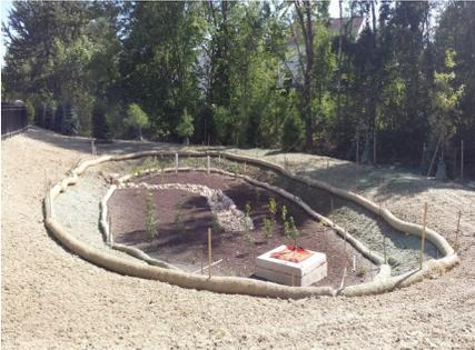
Bioswales are shallow, vegetated channels that slow down and infiltrate storm water runoff. Bioswales use an engineered soil sub-base made of topsoil, sand and compost. The vegetation and rocks in the trench reduce the velocity of the runoff and filter suspended sediments from the water. Bioswales are best suited along roadways and parking lots and sometimes act as pre-treatment devices for other storm water management practices.
