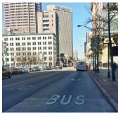
Bus only lanes are traffic lanes on a surface street that are restricted to buses either at all times or during certain hours of the day. Bus only lanes have signs posted along the route with specific regulations. Bus only lanes keep buses from getting stuck in traffic, improving the speed and reliability for bus riders and improving the overall traffic flow of a corridor. They are most appropriate in areas with very frequent service.
