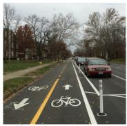
Two-way bike lanes are adjacent lanes accommodating opposite directions of bicycle traffic, striped onto the roadway next to the other travel lanes. They are sometimes installed in the middle of the street between travel lanes, but are more often at one side of the roadway. Two-way bike lanes must be designed properly to prevent safety hazards.
