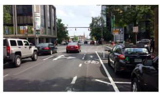
A bike lane is a portion of roadway that has been designated for preferential or exclusive use by bicyclists by pavement markings and, if used, signs. It is intended for one-way travel, usually in the same direction as the adjacent traffic lane, unless designed as a contra-flow lane.
