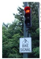
Bike signals are traffic signals designed specifically for bicycle traffic. Bike signals can improve traffic flow and reduce turning conflicts between bicycles and motor vehicles. For example, if a bike lane is to the right of a right-turn motorized vehicle lane, separate signals can instruct bicyclists and motorists to proceed (going straight or turning right) at different points in the signal cycle.
