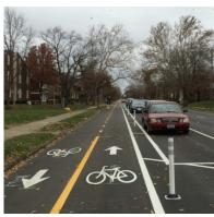
A protected bike lane (or cycle track) is an exclusive bike facility that combines the user experience of a separated path with the on-street infrastructure of a conventional bike lane. A protected bike lane is physically separated from motor traffic and distinct from the sidewalk. In situations where on-street parking is allowed, protected bike lanes are located to the curbside of the parking (in contrast to conventional bike lanes).
