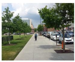
A sidewalk is a paved pedestrian path that is parallel and adjacent to the roadway. Sidewalk widths may vary, but typically are five feet, which allows two people – including wheelchair users – to pass comfortably or to walk side-by-side. They are measured in terms of "clear width" (the width that can be traveled freely, without obstacles). The clear width of a sidewalk does not include the area in which sign posts, street furniture, and other permanent or semi-permanent items are placed.
