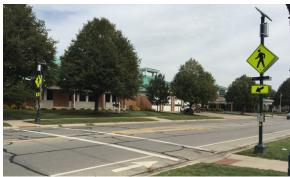
A signalized mid-block crosswalk is a signal that is activated by pedestrians when they want to cross the street. This can include pedestrian hybrid beacons (or HAWK), rectangular rapid flashing beacons (or RRFBs), and other treatments. Both types of beacons involve a push button trigger of flashing lights to warn motorists of pedestrians.
