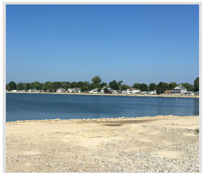
Buckeye Lake during reconstruction of the dam
