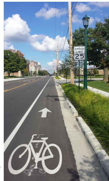
A bioswale curb in Upper Arlington buffers pedestrians from road users. Source: MORPC
