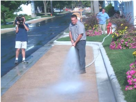
Permeable pavement in Canal Winchester allows rainfall to infiltrate the ground below. Source: MORPC
