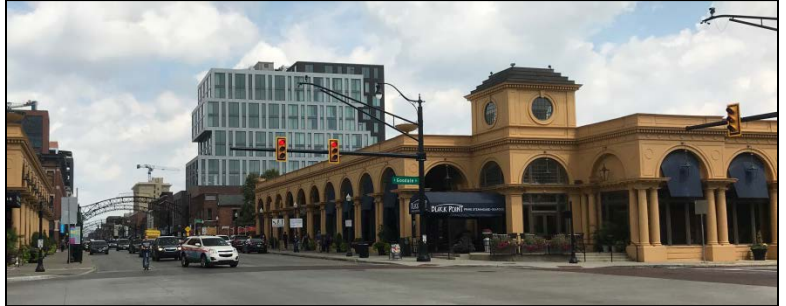
Figure 116 - High Street Cap over I-670.
