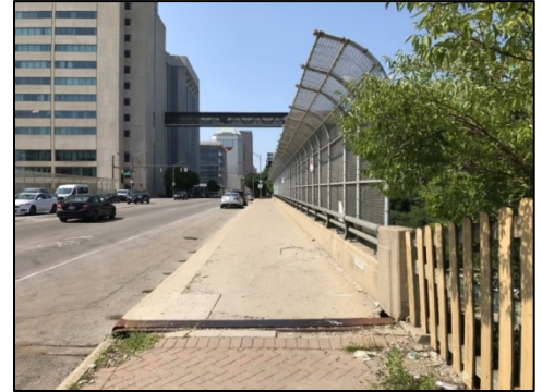
Figure 10 - High Street Bridge on eastern sidewalk of bridge (existing).
