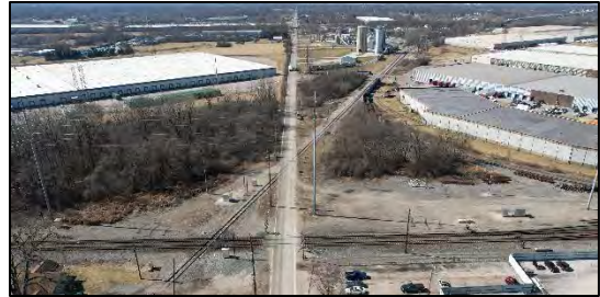
Figure 8 - The at-grade rail crossings with XPO Logistics (left) and ODW Logistics (right) in background.
