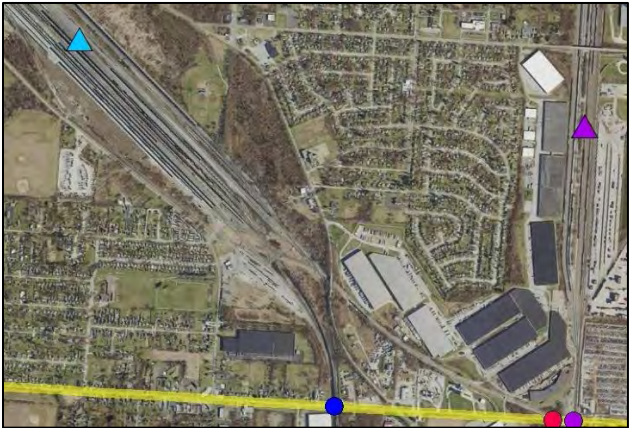
Figure 5 - Location of rail infrastructure. Parsons Yard is marked by a blue triangle, Watkins Yard by a purple triangle. Larger scale available in Appendix 2 - Williams Road Railroad Map .
