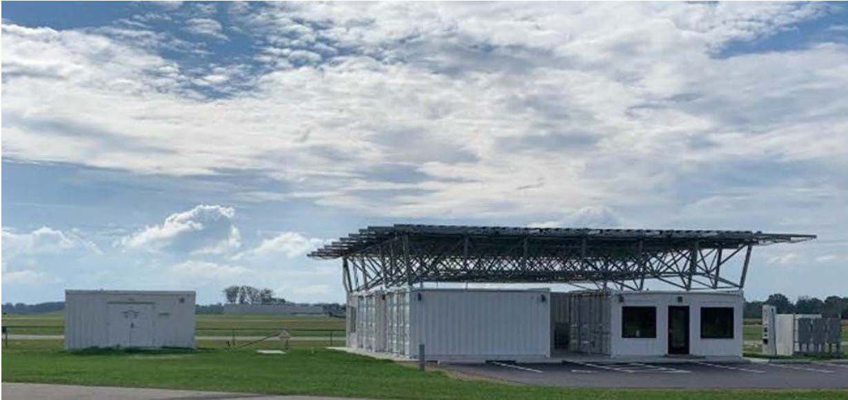
Vertiport at Springfield-Beckley Municipal Airport
