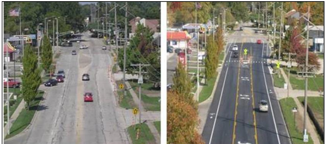
▲ Before and after a road diet. Note the addition of a center turn lane, bike lanes, and marked crosswalks. Champaign-Urbana, IL. (Source: Streetscape Improvements entry in the TDM Encyclopedia . Litman, 2011.)
