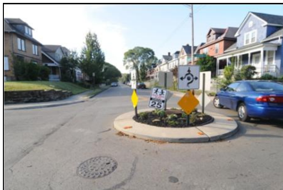
◀ A neighborhood traffic circle on E. Sycamore Street at Linwood Avenue. Columbus, OH. (Source: MORPC)
